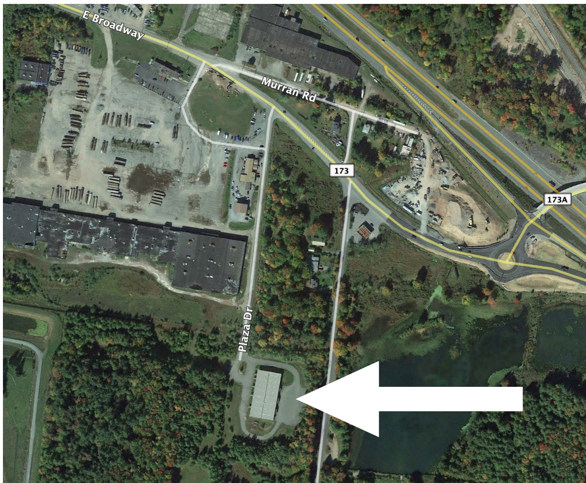
Aerial View of Existing Building/Site
